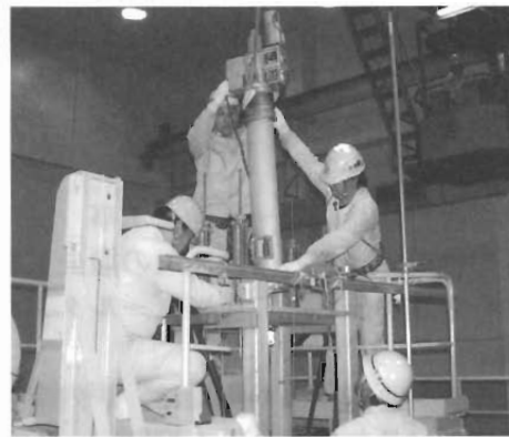
Photo10 Removal of Control Drive
