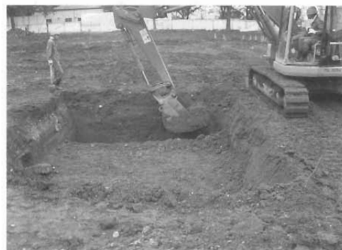
Fig.30 Digging the Ground 5\text{m}\times 5\text{m}
