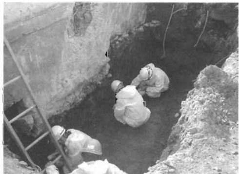
Fig.26 Contamination Survey at the Building Foundation
