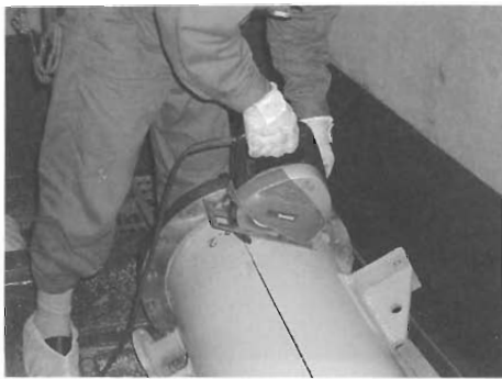
Photo17 Cutting of Demineralizer Tank
