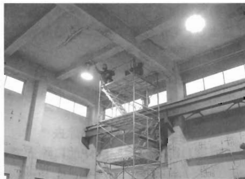
Fig.20 Contaminations Survey at the Wall with Rolling Tower Type Scaffolding
