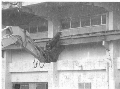
Fig.23 Removal of Crane Rail by Big Bite
