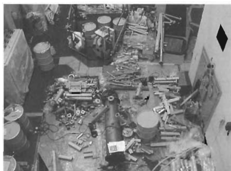
Photo21 Cutting of Equipment and Piping
