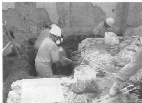
Fig.11 Removal of Pipe Under Ground
