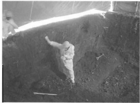
Fig.24 Search and Removal of the Materials Under Ground
