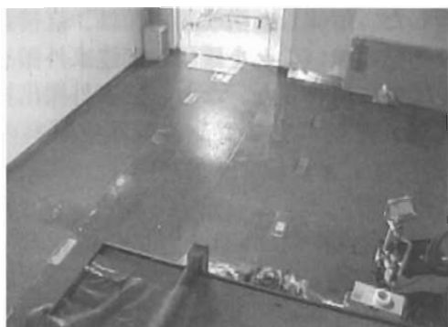
Photo 4 Situation after Semi-Hot Cell Removal
