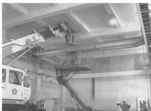
Fig.14 Dismantling of Crane
