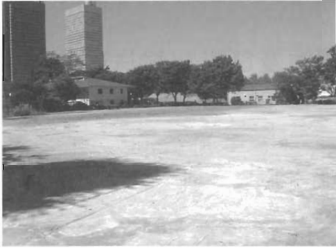
Fig.35 Over View of Clear Site Filled with New Soil Mud.
