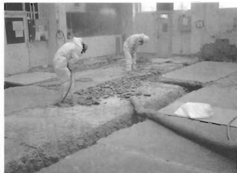
Fig.10 Concrete Removal by Breaker
