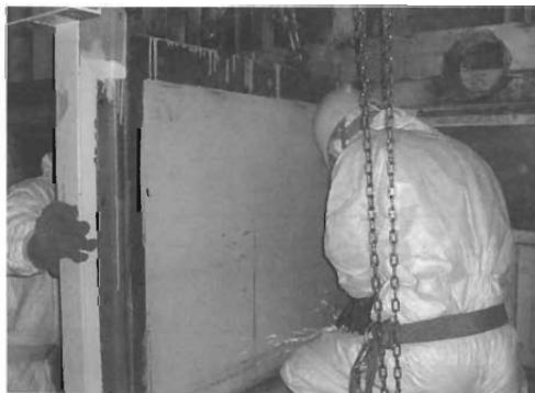
Photo 5 Dismantling Work of Partition Plate between the Junior Cells
