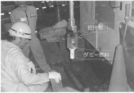
Photo 4 Mock-up Test of Tool
