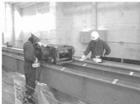
Fig.15 Contamination Survey for Removed Crane Beam
