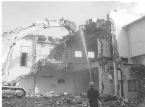
Fig.22 Dismantling of Buildings, Water Spray Applied
