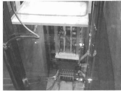
Photo 9 Reactor Core Seal Plate
