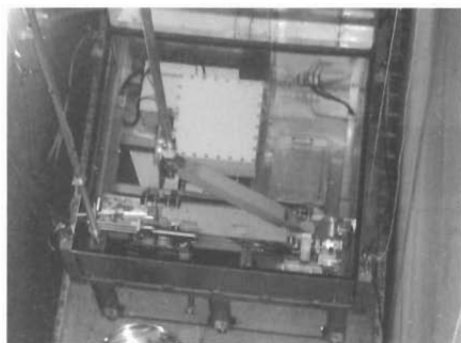
Photo 1 Underwater Equipment for Fuel Handles Cutting
