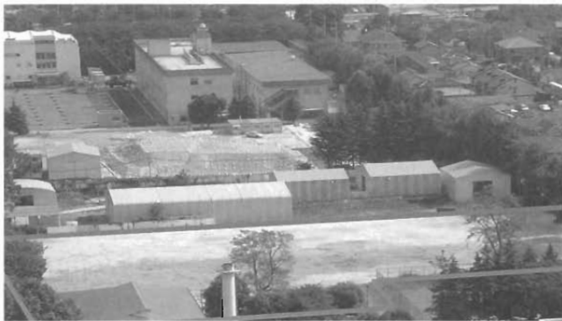
Fig.36 Over View of Nuclear Institute. Site after Decommissioning at 2003/10/1
