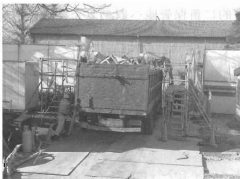
Fig.32 Survey on the Car and Materials Before Carrying Out
