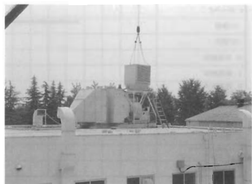
Fig.6 Dismantling of Fan and Filter Unit at Roof
