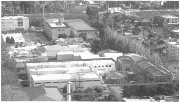
Fig.1 Over View of Nuclear Institute. Before Decommissioning at 2003/1/10
