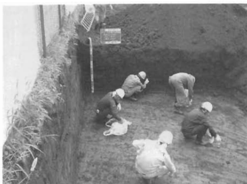
Fig.31 Contamination Survey at the Depth of 0m, 0.5m, 1.0m, 1.5m
