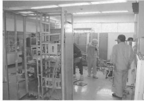
Photo15 Dismantling of Instrument and Control System in Control Room
