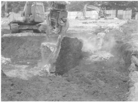
Fig.27 Removal of the Building Foundation for Contaminations Survey
