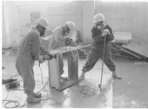
Fig.7 Disassembling of Filter Unit in the Building
