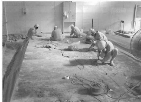
Fig.9 Strip Paint for Radioactive Contaminations Survey on Concrete Surface
