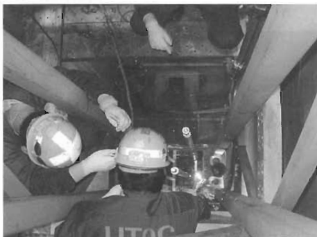
Photo12 Withdrawal of Reflector Element
