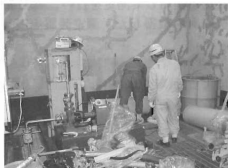
Photo16 Dismantling of Pool Water Clean-up System
